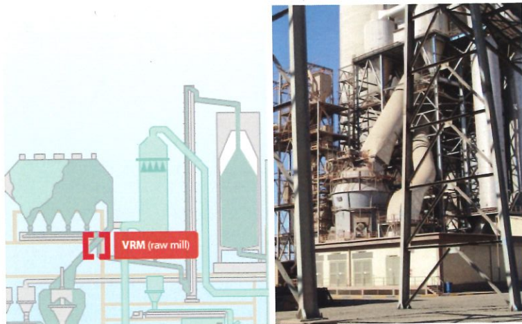
Raw mill application.
